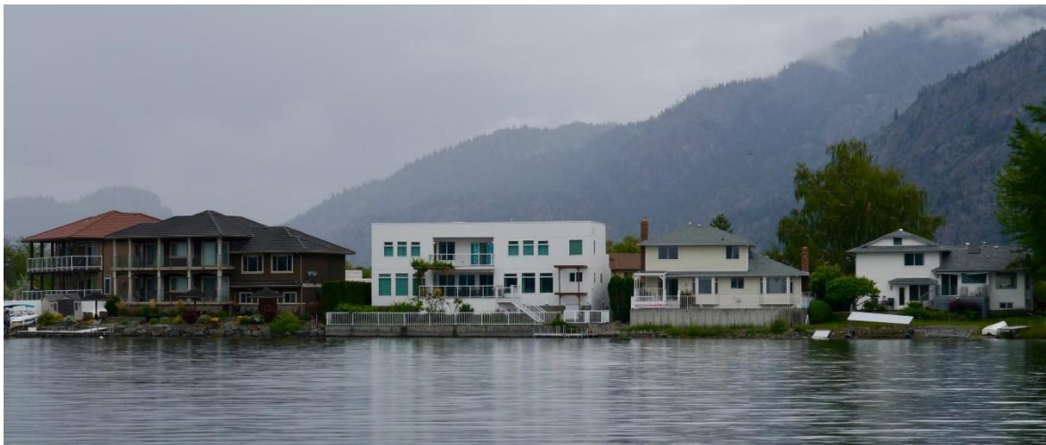
Shoreline development with erosion control structures on Osoyoos Lake, May 2019
