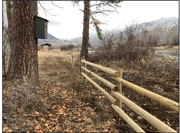
Portion of new SILT boundary fence
