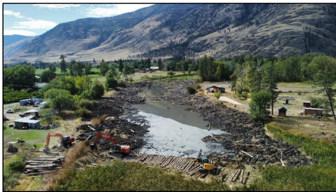
Phase 2 excavation near complete
