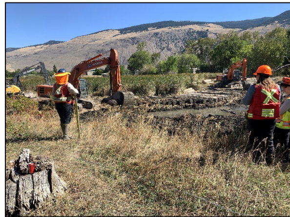
Phase 2 excavation in progress
